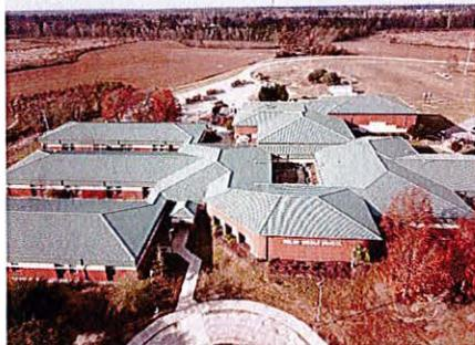
Both projects consisted of metal roof retrofits over existing membrane roofs. They required the demolition of skylights and related interior renovations to lighting and suspended ceilings, re-routing of mechanical elements, as well as some site utility work to accommodate the roof drains.
