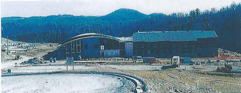
Watauga High School under construction, March 2009
