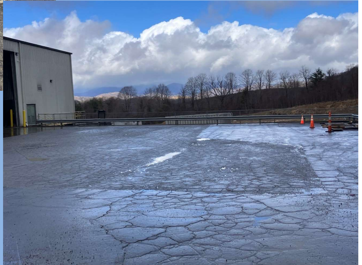
Pavement at commercial entrance
