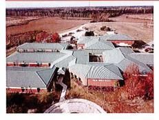
Both projects consisted of metal roof retrofits over existing membrane roofs. They required the demolition of skylights and related interior renovations to lighting and suspended ceilings, re-routing of mechanical elements, as well as
