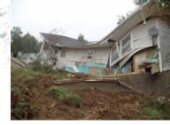
2004 – A modified slope failure at the White Laurel Subdivision resulted in severe damage to numerous structures. (Left)
